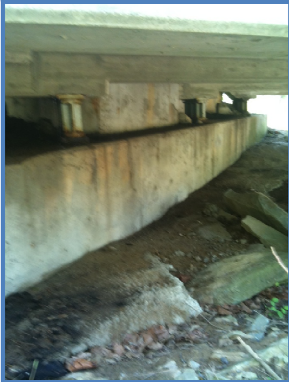
Rockers at East end of the Bridge
