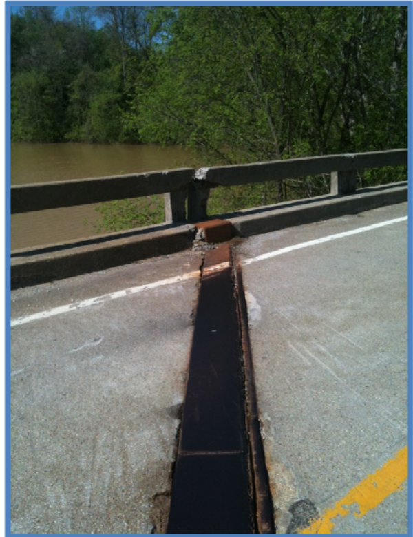
Steel Sliding Plate Expansion Joint
